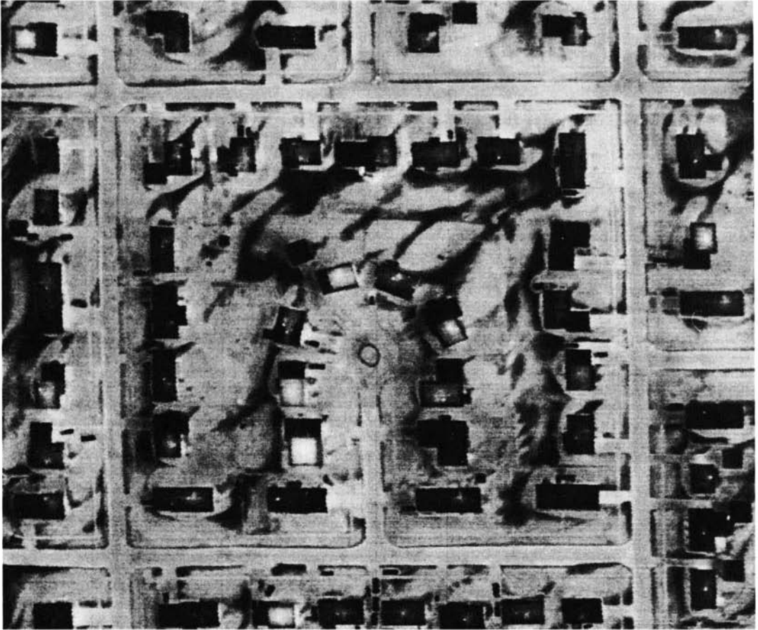
Figure 5.22 Nighttime thermal image depicting building heat loss in an Iowa City, approximately 2:00 A.M., snow-covered ground, air temperature approximately -4^{\circ}\text{C} , 460 m flying height, 1 mrad IFOV. (Courtesy Iowa Utility Association.)
