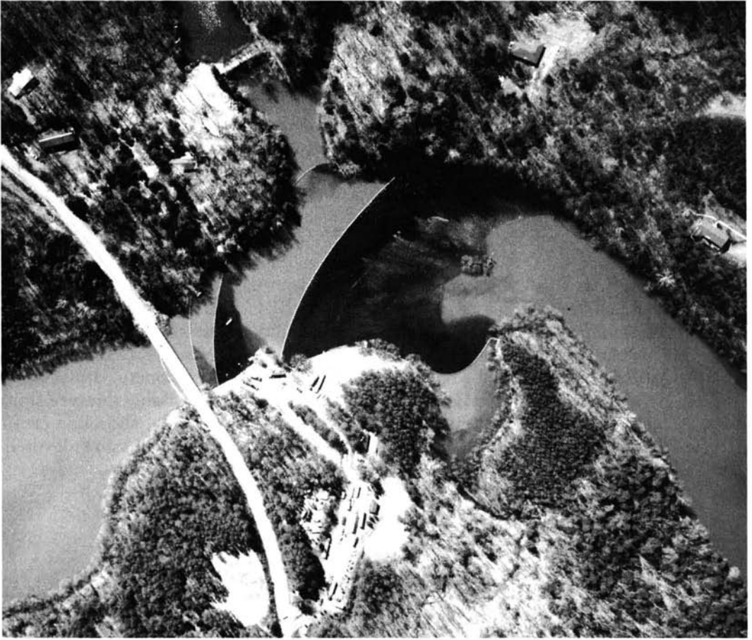
Figure 4.43 Aerial photograph of an oil spill on Bull Run, near Manassas, Virginia. Note the series of booms placed across the river to entrap the oil (the flow of water is from right to left in this photograph). (Courtesy EPA Environmental Photographic Interpretation Center.)
